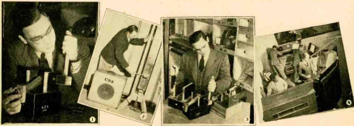
1.—The "squeak box," WOR's latest. It can produce any squeak from the sound of a pair of Caspar Milquetoast shoes to the swinging of a heavy castle gate. The turning shaft, leather belt and adjusting screw are easily seen in the picture. 2.—Thunder from the studio. The sound man strikes a tympani mallet against a sheet of metal wired to an amplifier. 3.—Three of the new "squeak boxes." The center one is the latest edition, used on such shows as "Murder Clinic," "Highway Patrol," "Nick Carter," "Superman" and others. 4.—A staff of four sound-men were required to handle the effects during the dramatization of a bombing mission to Hamm, Germany, aboard the Flying Fortress, "Stormy Weather."
